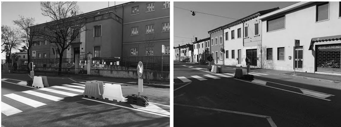
Figure 17 - Positioned crosswalk island
